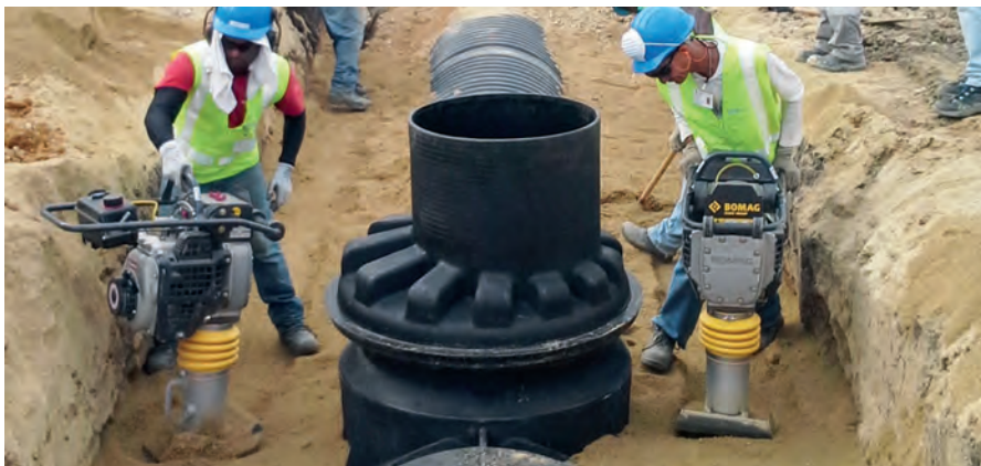
▲ Wastewater-transfer network in the Dominican Republic.
