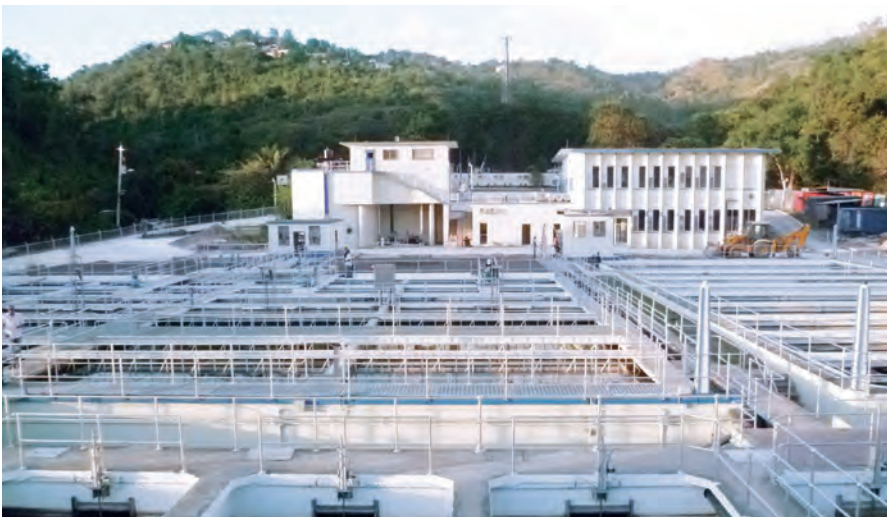
▲ Constant Spring Water Treatment Plant, Kingston, Jamaica.
