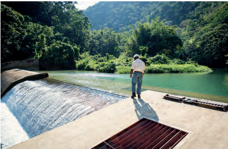
▲ Hope River intake structure in Jamaica.
