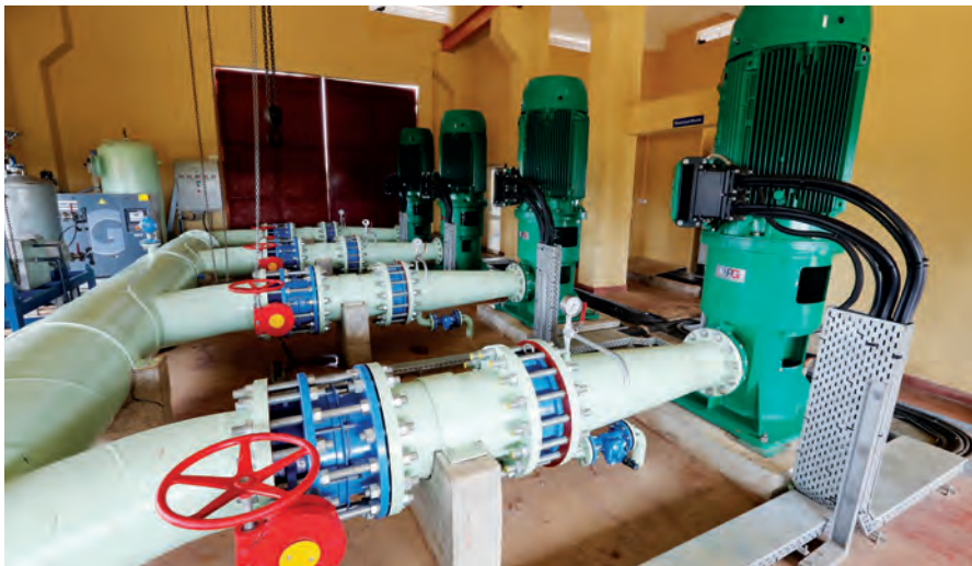
▲ Kantale Pumping Station, Trincomalee, Sri Lanka.
