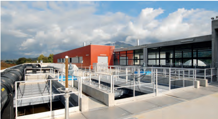
▲ Campo Dell'Oro wastewater treatment plant in Ajaccio, Corsica, France.
