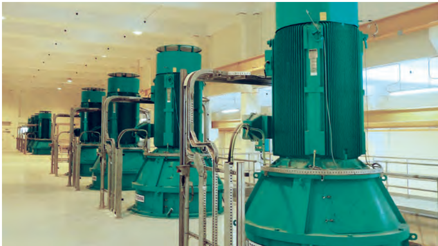
▲ Doha North Pumping Station (PS70), Qatar.
