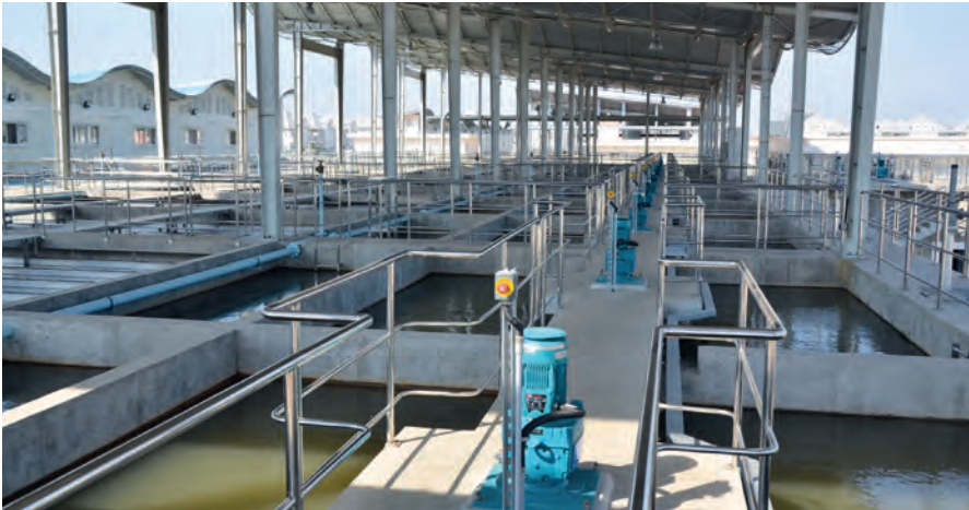
▲ Niroth Water Treatment Plant, Phnom Penh, Cambodia.
