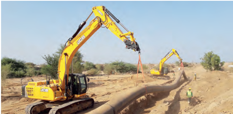
▲ Drinking water transfer network in Djibouti.
