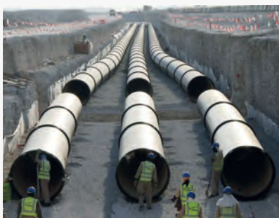
◀ Pumping mains, Doha North Pumping station (PS70), Qatar.
