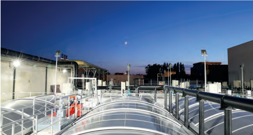
▲ Brussels South wastewater treatment plant in Belgium.
