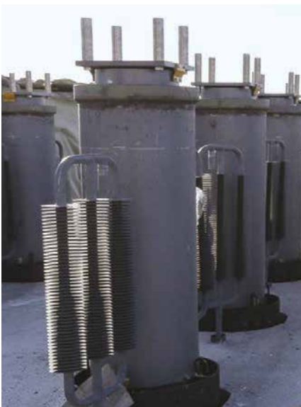
Innovative pile design in the permafrost
