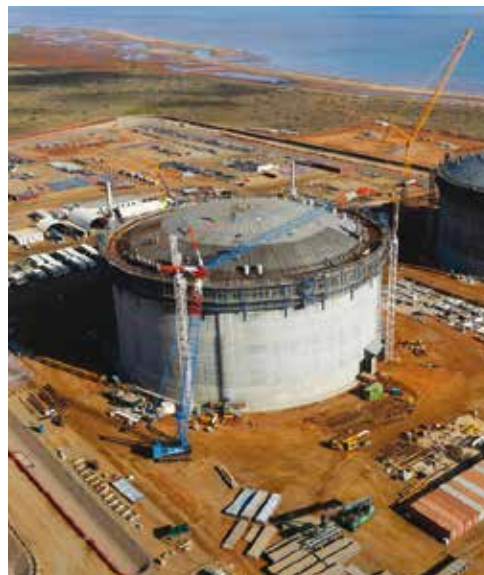
Self-climbing formwork in remote warm region
